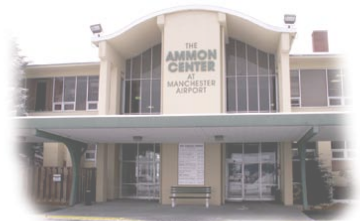
OTIEC/Region 1 at Manchester/Boston Airport • 175 Ammon Drive • Manchester, NH
